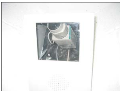
Camera in high-risk cell faces ceiling. Tohono O’odham, AZ
