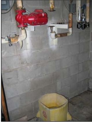
Missing pump/leaking water. Medicine Root Jail, SD
