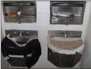
Inoperable sinks in cells. Mescalero, NM
