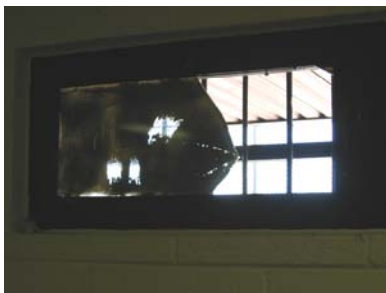
Broken glass in cell window. Hopi, AZ
