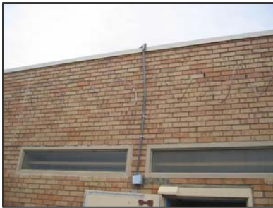
Electrical conduit used to escape. Medicine Root, SD
