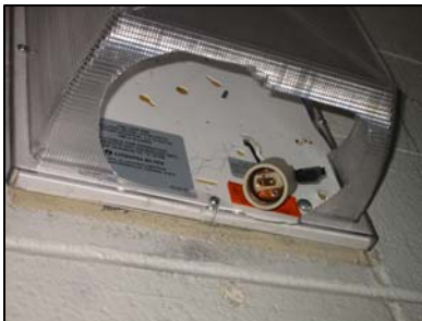
Broken light fixture observed during May 2004 Yakama site visit.
